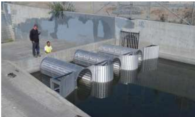
City of Milpitas Storm Flo Screen (photo courtesy of Roscoe Moss Company)
