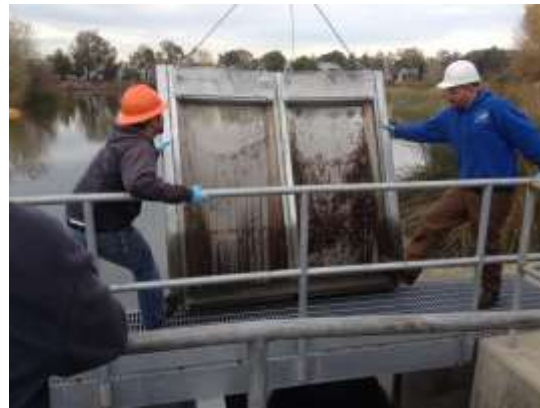
(Cleaning operations at the City of Santa Clara pump station)
