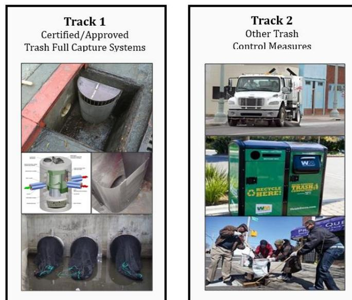
**Figure 4.** Examples of Track1 and Track 2 control measures.
